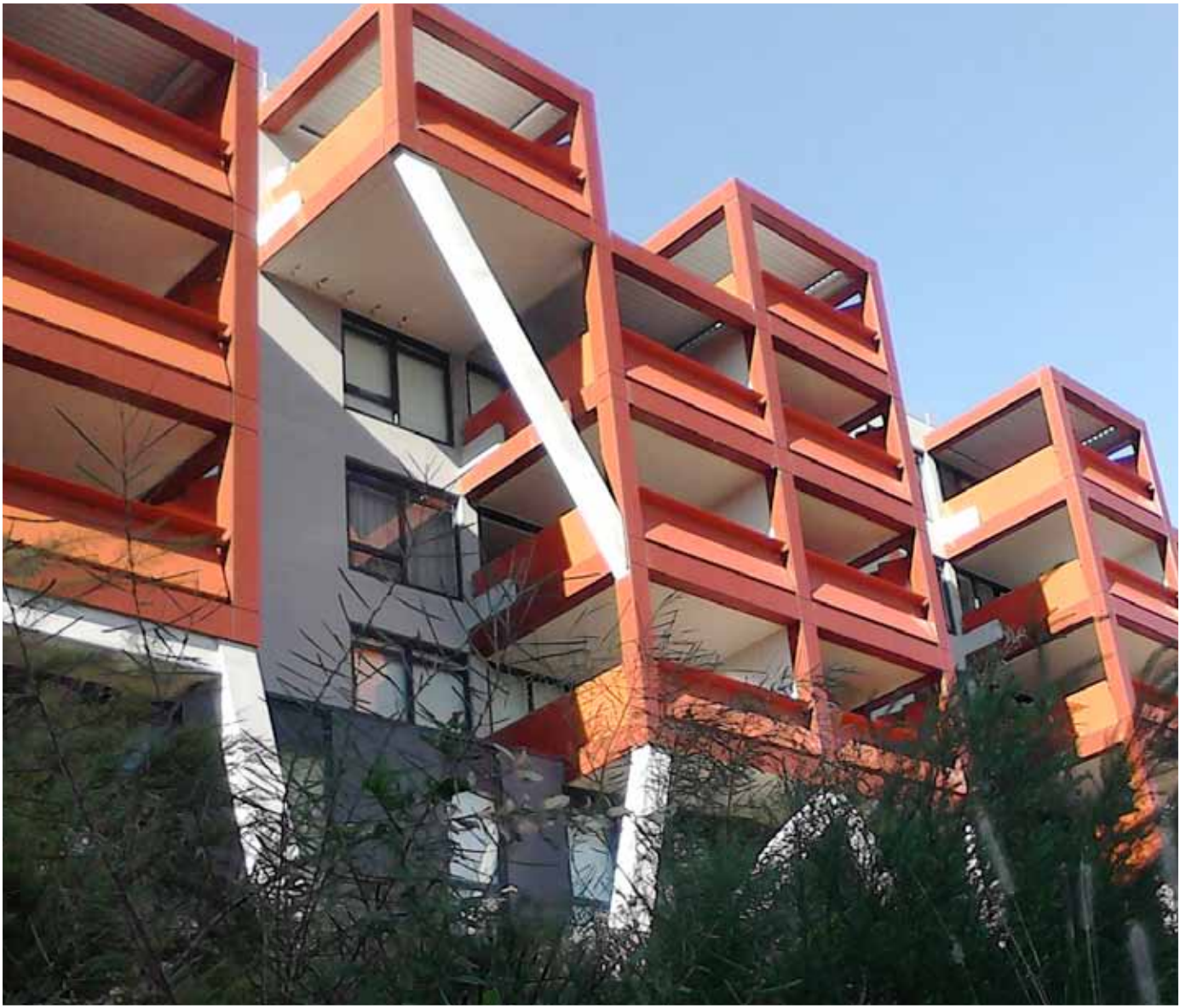
Antias Building in the Jackson's Landing development, Pyrmont Source: photograph by Dr Alasdair Jones
